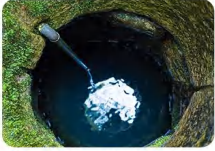
DEEP WELL WATER INTAKE
