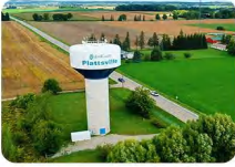
WATER TOWER WATER SUPPLY
